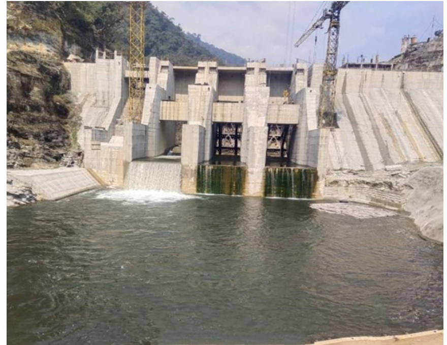
Dam works – River diverted through Radial gates
