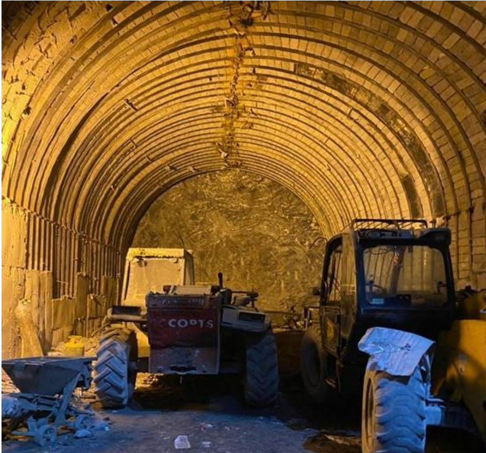
Horizontal Penstock Excavation
