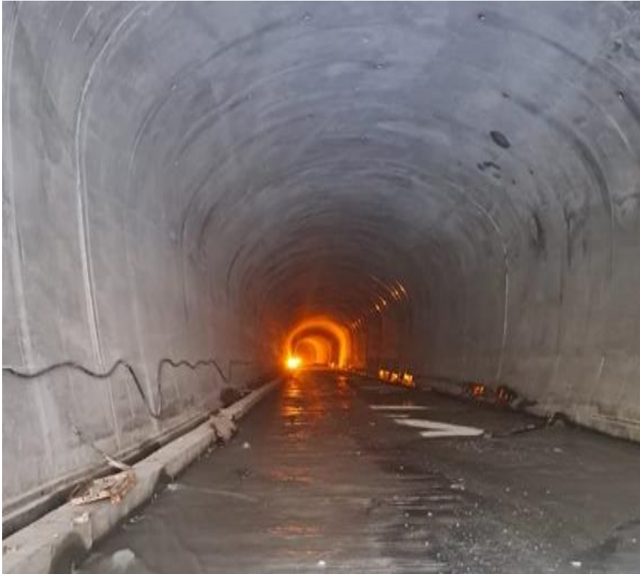
Tunnel invert lining
