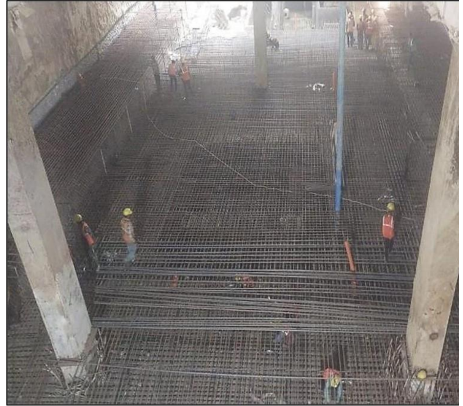
Station Base slab works Grid 5-8
