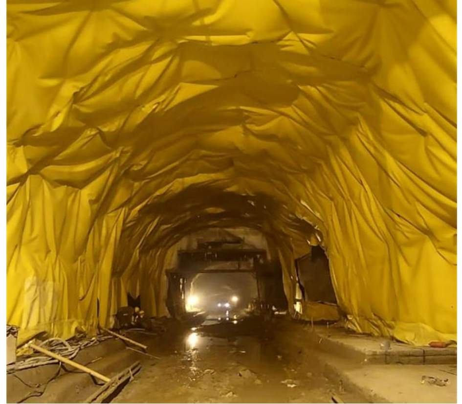
Escape Tunnel Layby Water Proofing Membrane fixing
