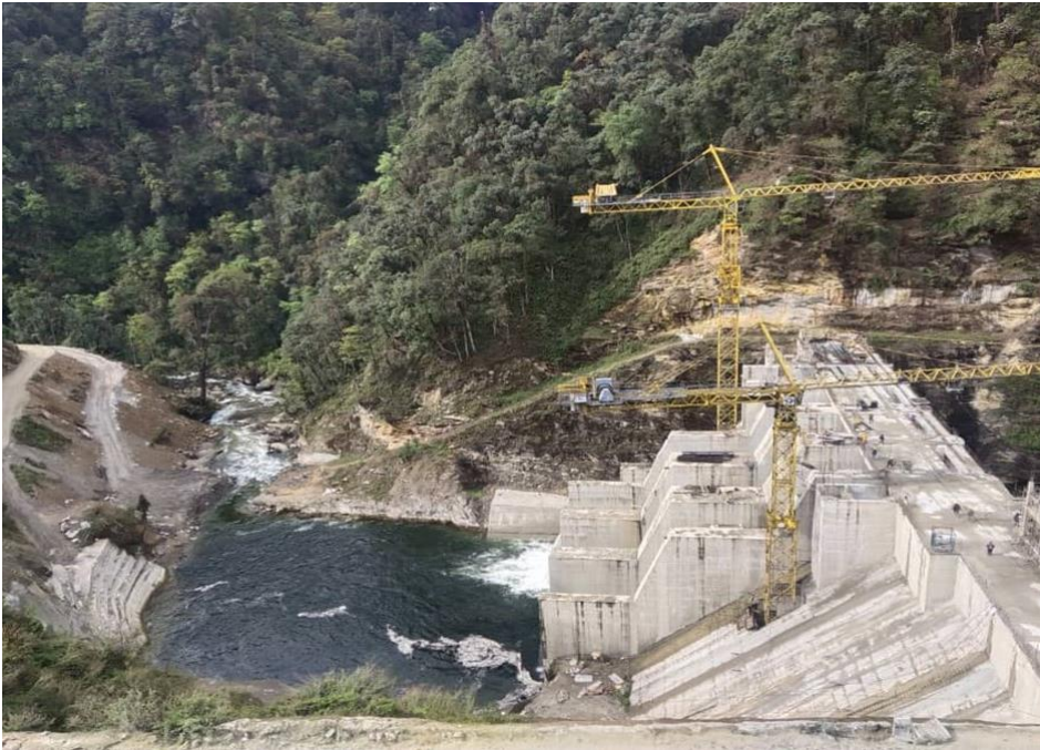
Dam works – River diverted through Radial gates
