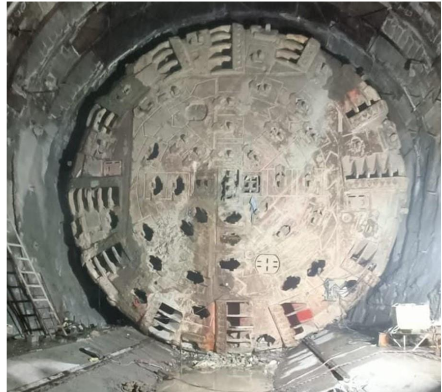
TBM Cutter Head
