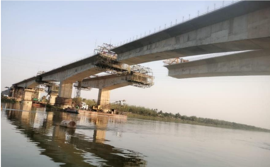
Bhagirathi bridge super structure works
