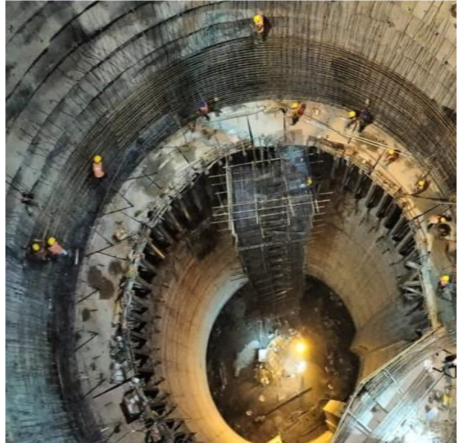
Downstream Surge Shaft Lining
