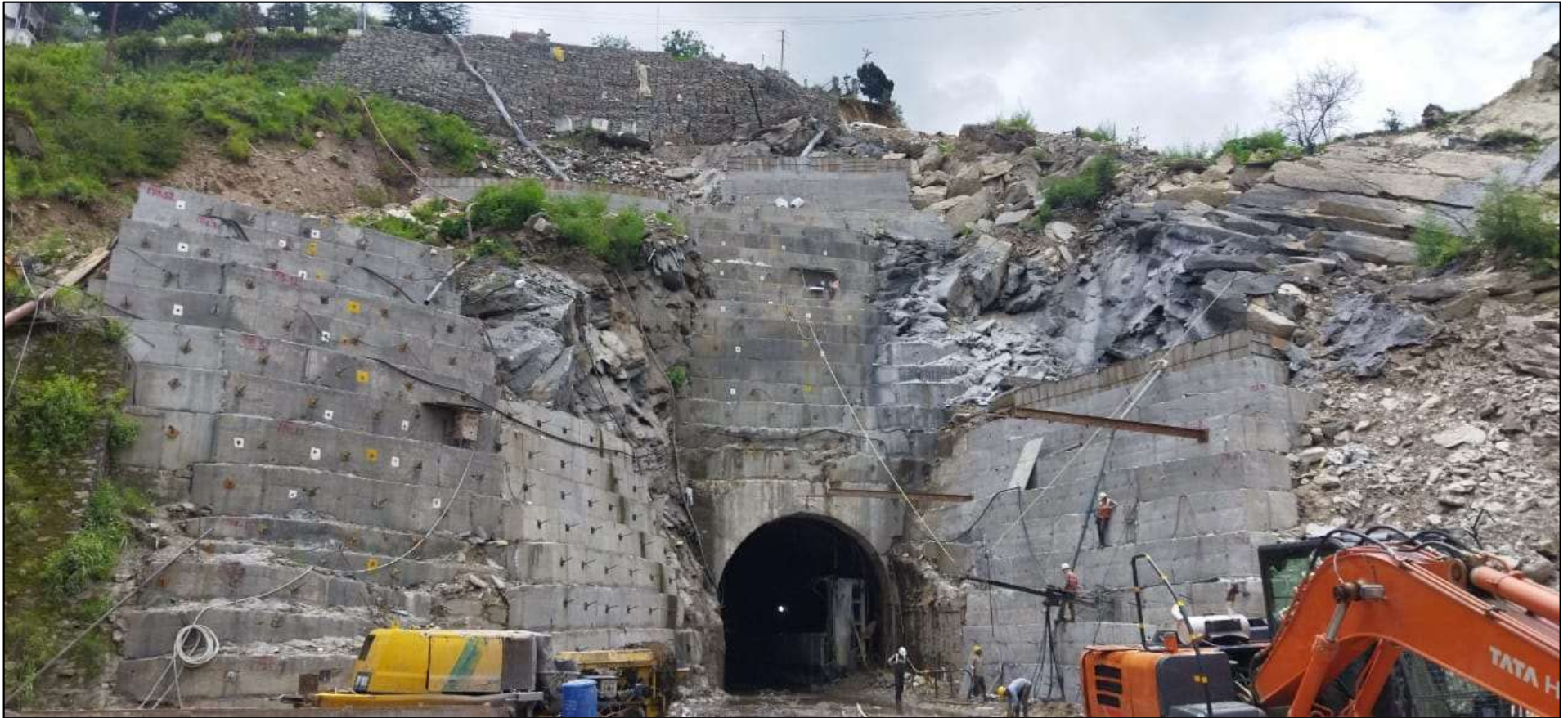
Restoration of TBM Portal
