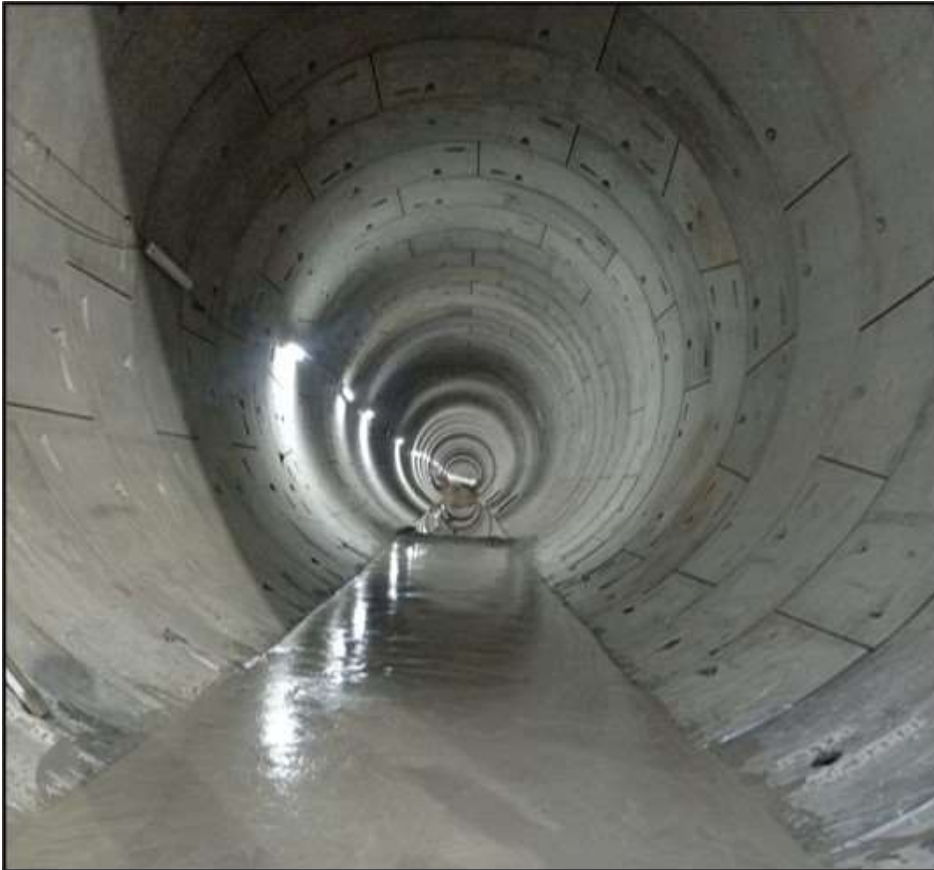
Invert Concrete Completed up to 70 Rm
