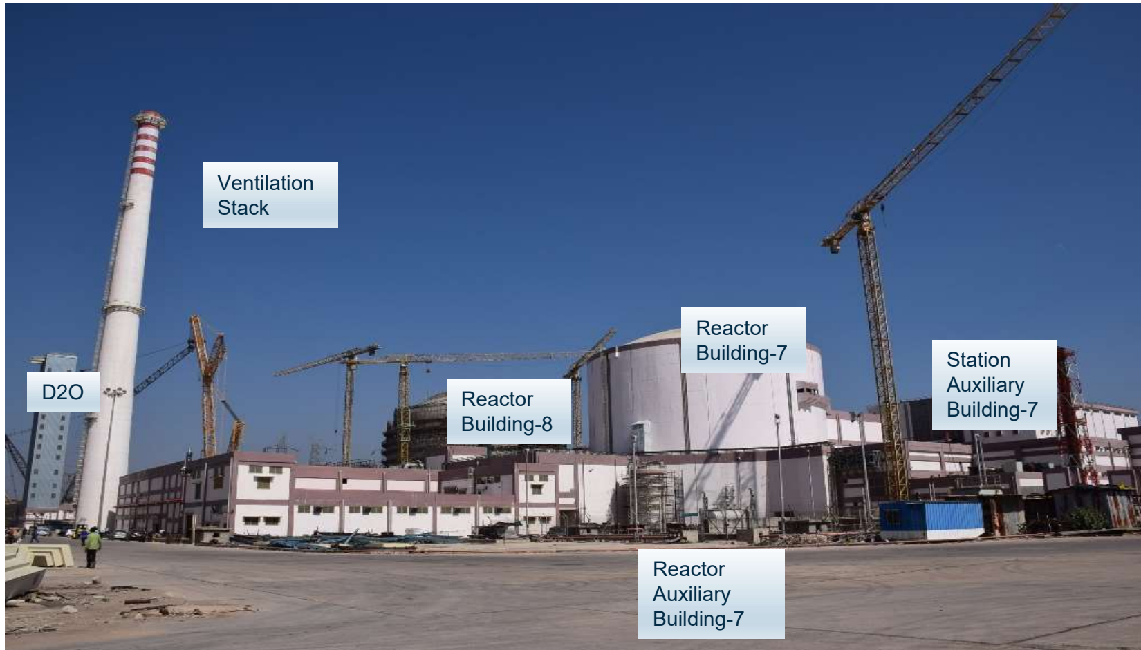
RB-7 & RAB-7, WMP, Ventilation Stack & D2O
