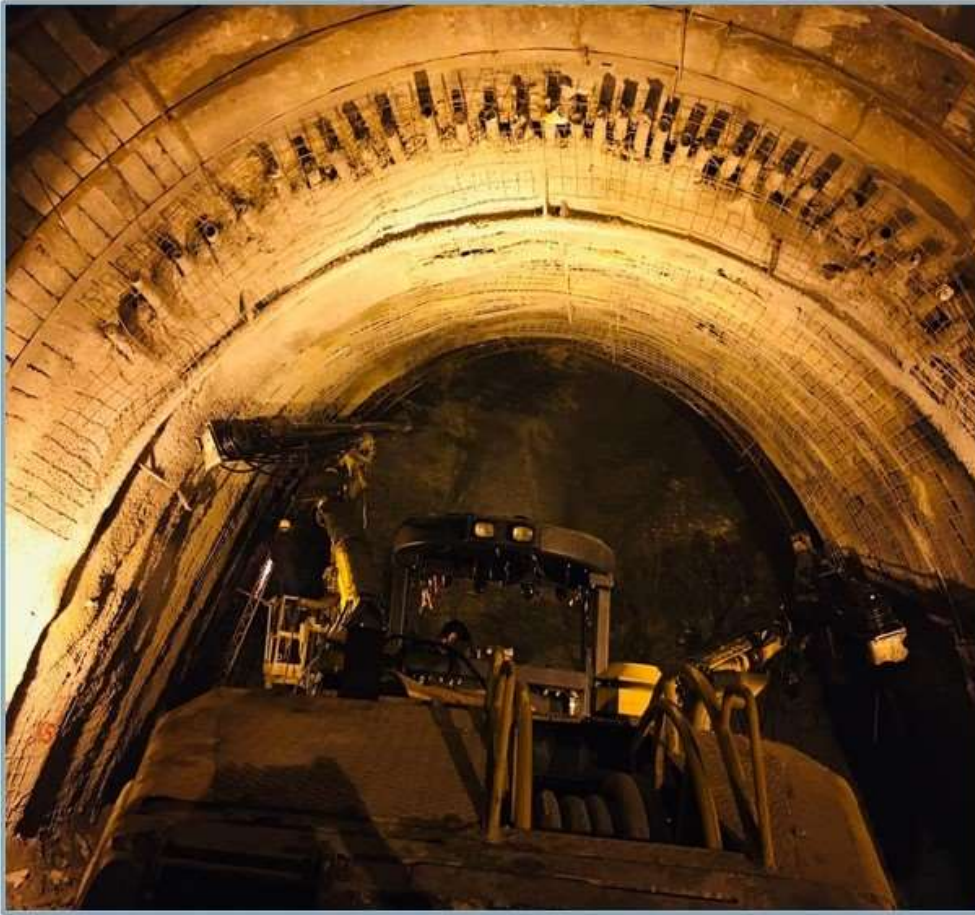
TBM Entry Adit Lattice Girder Fixing
