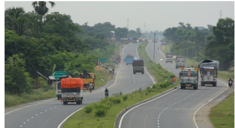
Km 341 (Farakka Raiganj Highway)
