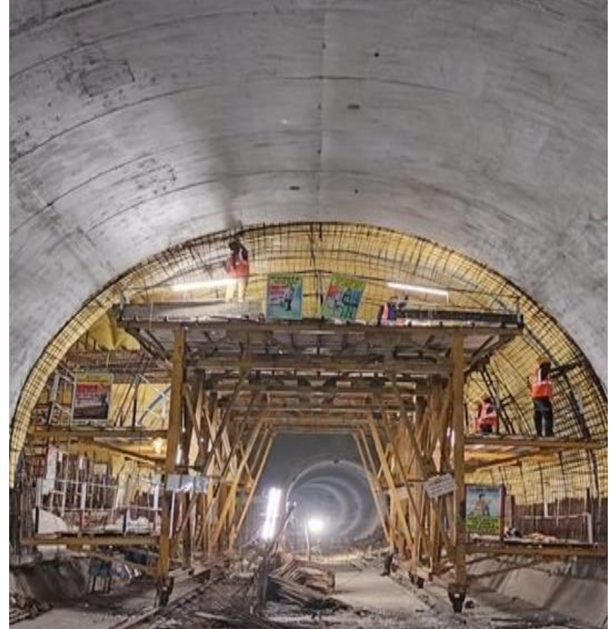
NATM finishing works in progress.
