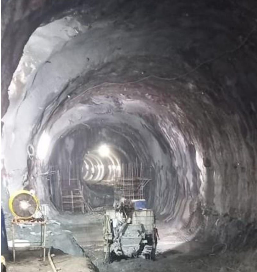
NATM benching works in progress.
