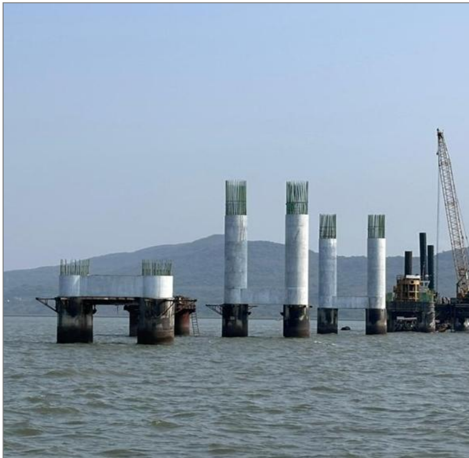
Pile, Crossbeam and Pier between P30 to P33
