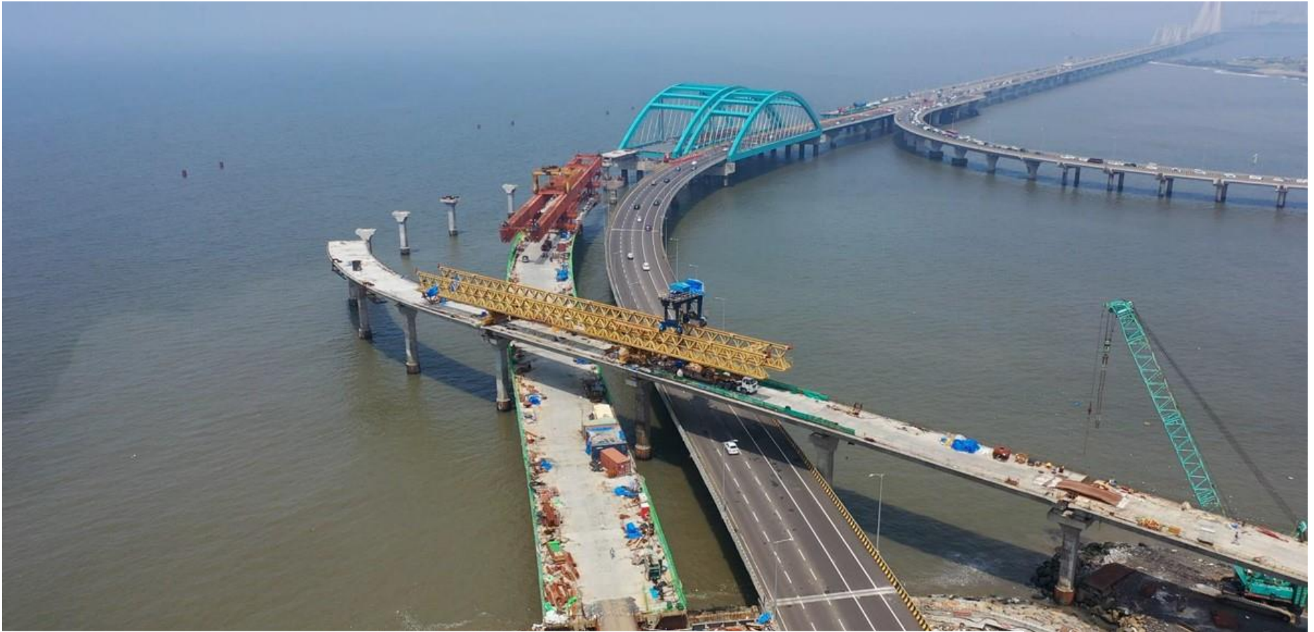
Main Bridge Segment Launching works
