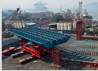
The first navigation span of the composite bridge was successfully launched on between the piers on February 02, 2024.
