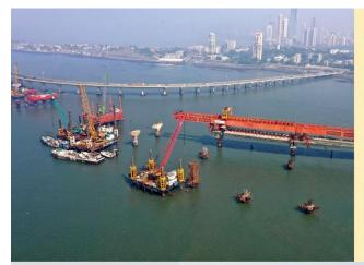
All monopile foundation work has been completed. Monopile help reduce total piles from 424 to 79. This is the first large scale monopile implementation in India.
