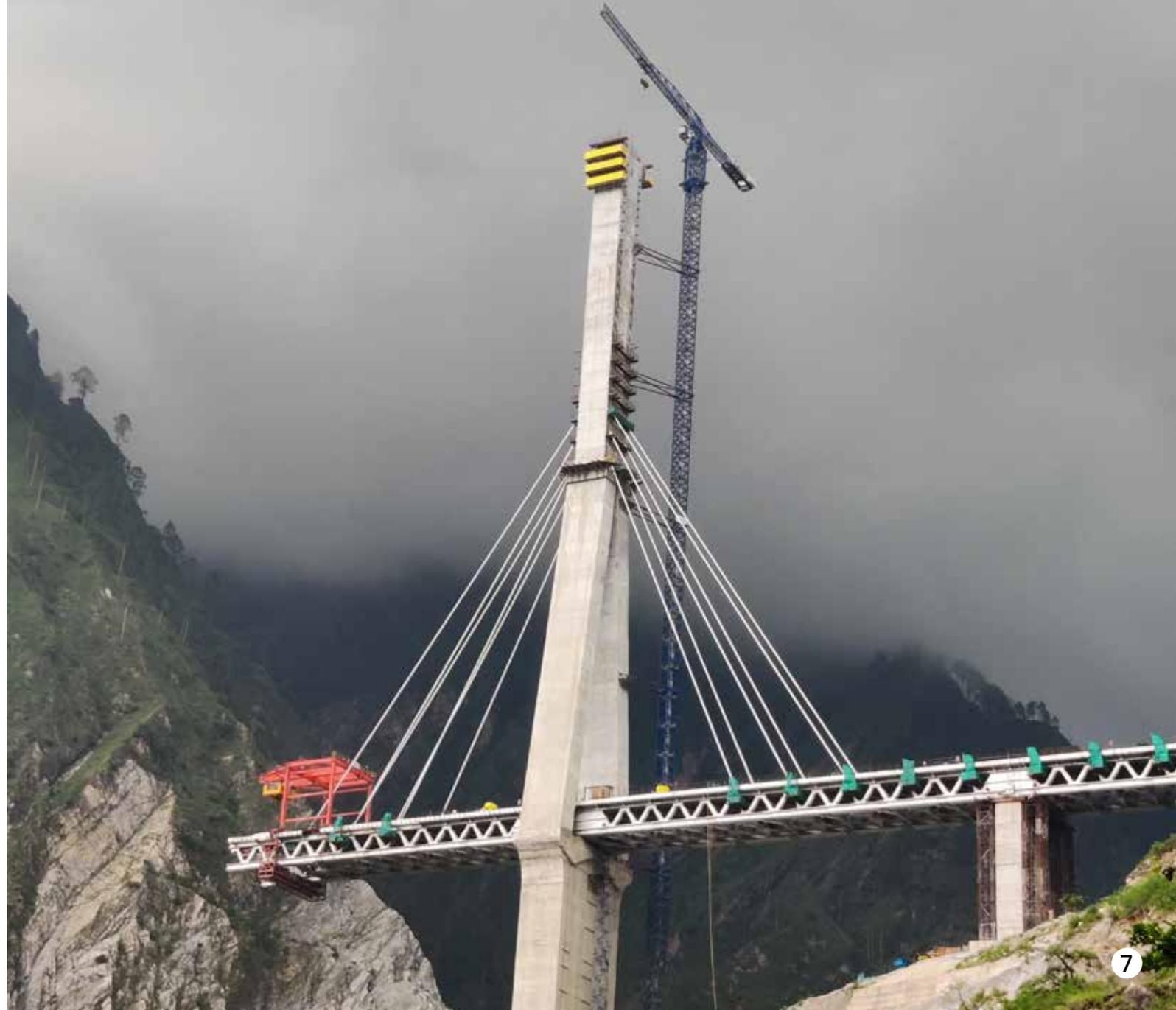
**7. Anji Khad Bridge:** The Main pylon construction of India's 1<sup>st</sup> cable-stayed rail bridge is completed, and 196 m deck slab finished out of 477m. Entire fabrication of approx. 8,000 MT was carried out at workshops in Gujarat and were shifted to the project site in trailers. Around 400 trailers travelled on the shoulders of the Anji gorge to reach the project site.
