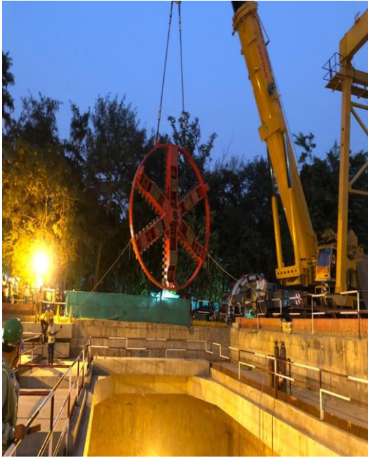
DMRC DC-06 Tunnel Boring Machine 5.8 m dia
