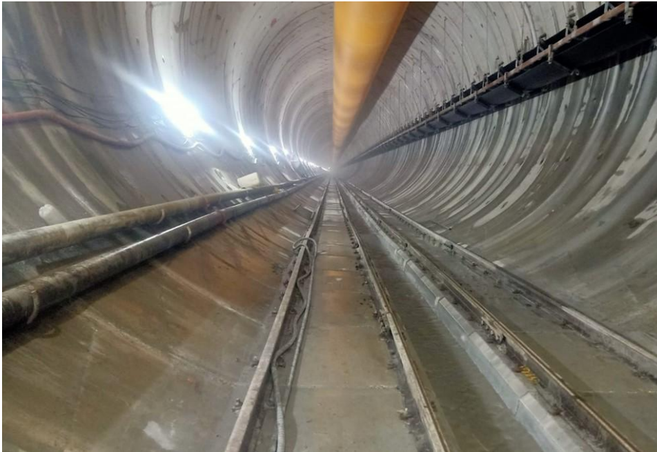
HRT by TBM
