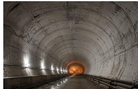
Tail Race Tunnel
