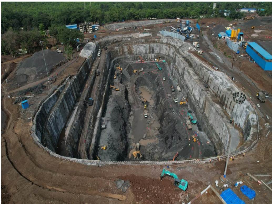
Powerhouse Excavation
