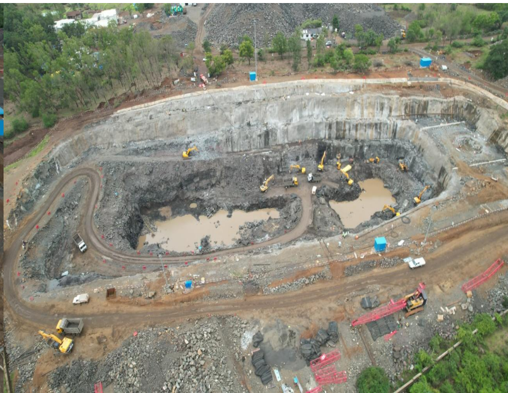
Upper Intake Excavation
