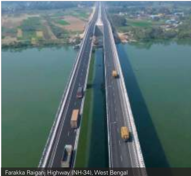
Farakka Raiganj Highway (NH-34), West Bengal
