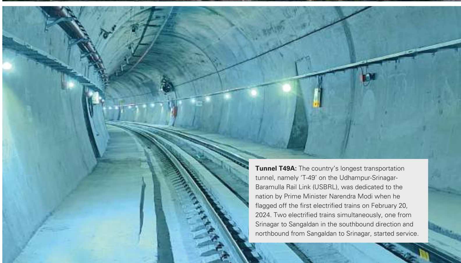
Anji Khad Bridge: The construction of the first cable stay bridge of Indian Railways in J&K along the Indian Railways' 356 km Jammu – Baramulla line was completed in September 2023. Key milestones included the completion of the Ancillary Viaduct, Central Embankment, final stressing of cables and track laying. Approach road, slope stabilization, and other miscellaneous works are underway.
