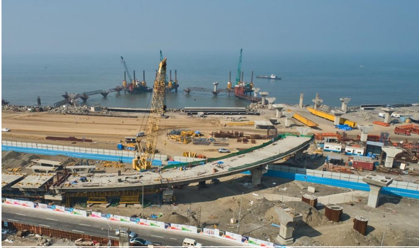
Arm 2 - Segment Erection
