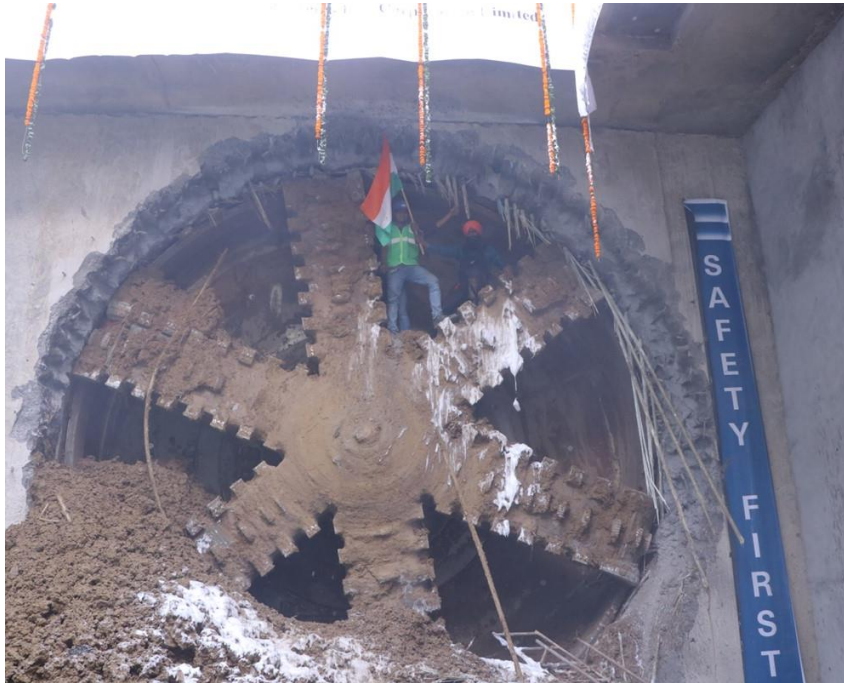
Tunnel Breakthrough-Upline
