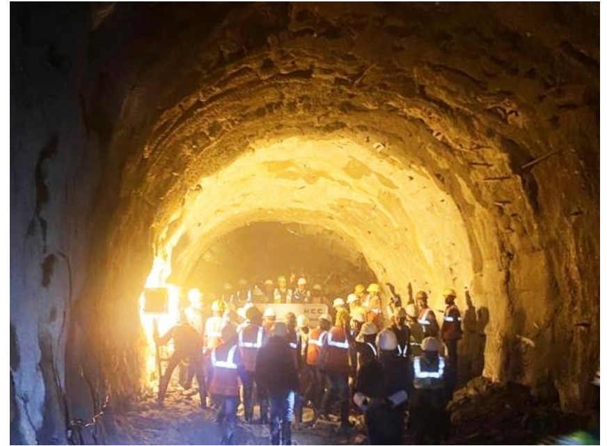
HRT Excavation completed
