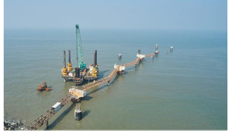
Arm 3 - Marine Piling
