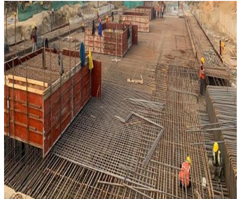
Station Roof slab in progress
