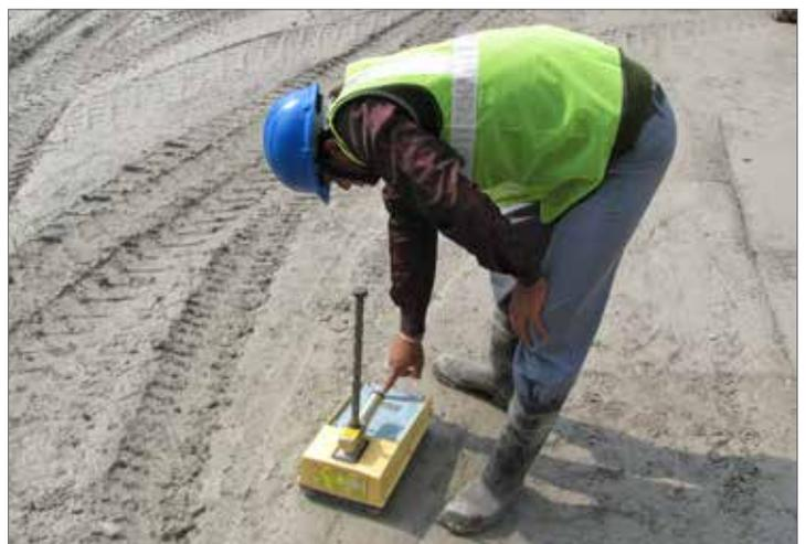
1) The heavy steel shuttering for the dam was placed at the precise location with the help of Hydra's and Tower Crane. 2) The RCC mix is carried to the required location by dumpers and spread in a 300mm thick layer using dozers. 3) This layer is then compacted using ten ton vibrating rollers. 4) The compacted concrete is tested for its density with a special device called 'Nuclear Density Gauge'
