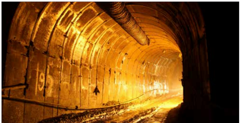
Additional supports provided at the access tunnel due to poor geology
