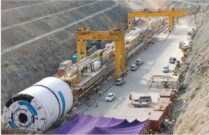
Largest diameter (10 M) Tunnel Boring Machine deployed at Veligonda Tunnel
