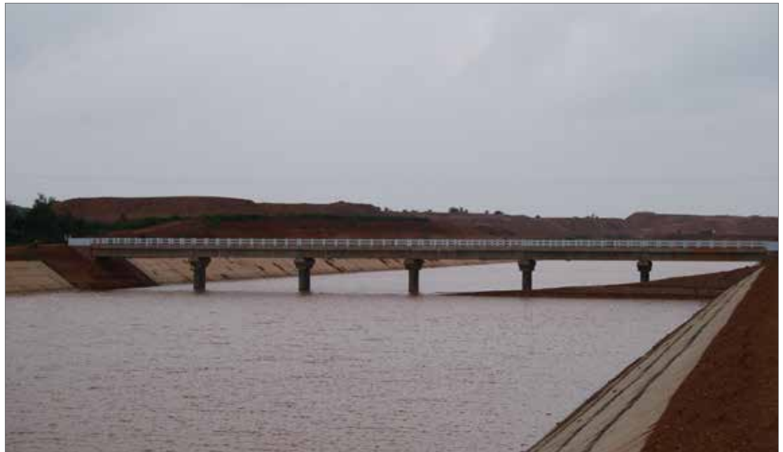
The 30.712 km long package 3 of the Polavaram Right Main Canal, part of National River linking project
