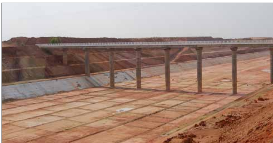
Deep Cut reaches at the Polavaram Canal yes
