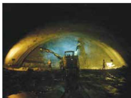
The powerhouse crown done by full face drill & blast
