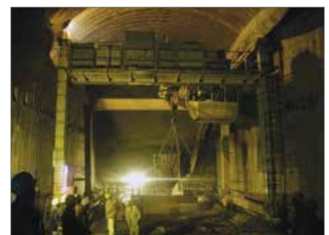
Powerhouse roof supported by lattice girder
