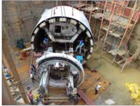
The TBM is lowered in the shaft piece by piece and assembled for the drive towards Shalimar Bagh Station
