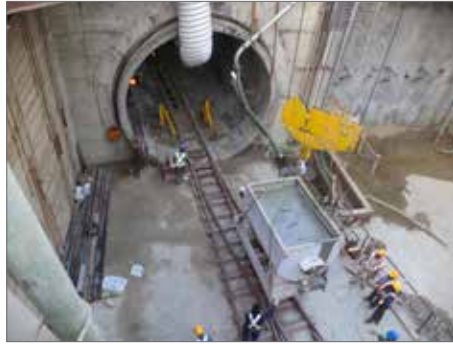
Concrete slurry being sent inside the tunnel
