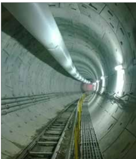
Finishes section of the up-line tunnel
