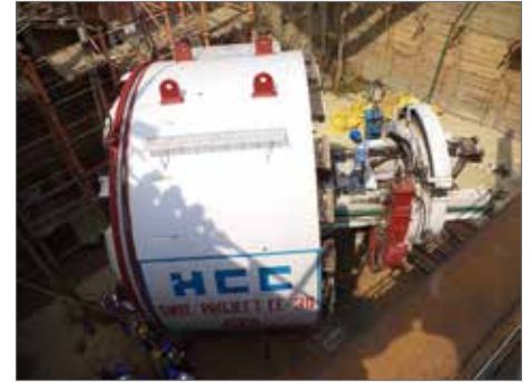
The TBM is lowered in the shaft piece by piece and assembled for the drive towards Shalimar Bagh Station
