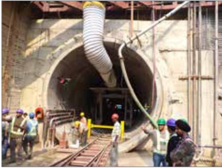
TBM begins the drive from the shaft area
