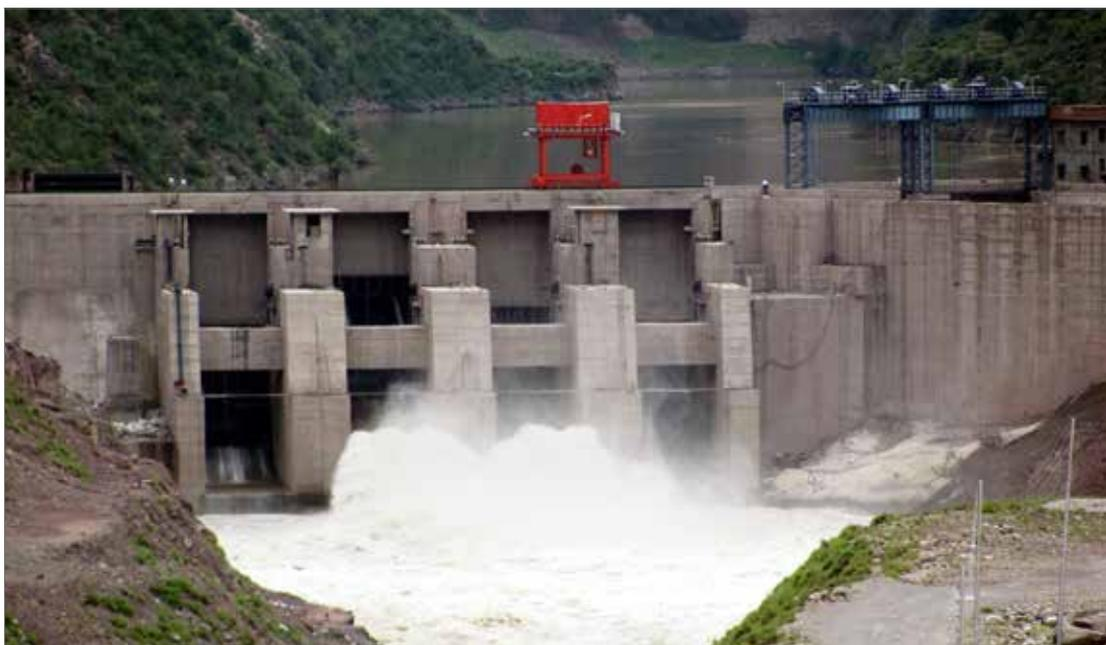
A downstream view of the 52 m high concrete gravity dam at the Uri-II HEP on River Jhelum in Jammu and Kashmir
