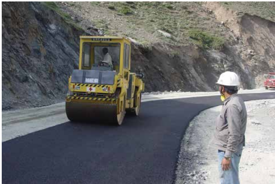
Asphalting work in progress at Shopian Sector of the Mughal Road
