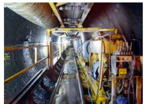
day with one tunnel boring machine, and a maximum progress of 543 m was achieved in a month. After completion of the tunnel boring, a concrete lining was provided, to give the tunnel a finished diameter of 3 m.
