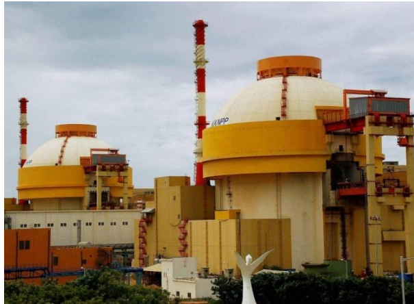
Kudankulam Nuclear Power Plant
