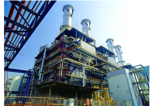
Uran Gas based Power Plant, Trombay
