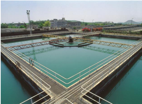
Bhandup Water Treatment Plant, Mumbai
